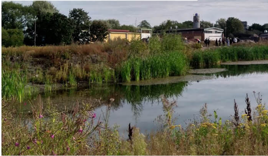
Wastewater treatment area
