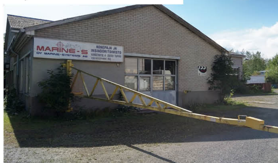
Repair and metalworks
