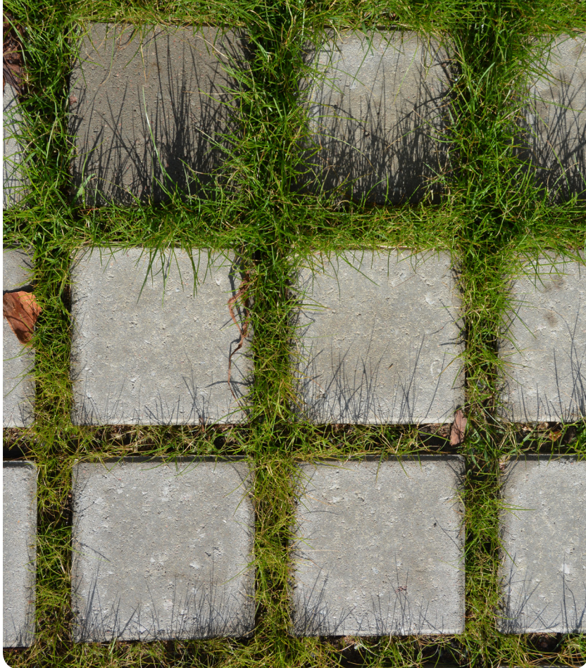
Grass, for example, can grow between permeable paving slabs. Photo: Aino Saarinen
