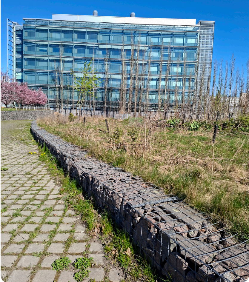
Stone gabions are low-maintenance, weather-resistant and long-lasting solutions. The stone gabion pictured is located in Viikki, Helsinki. Photo: Hilja Kurkinen
