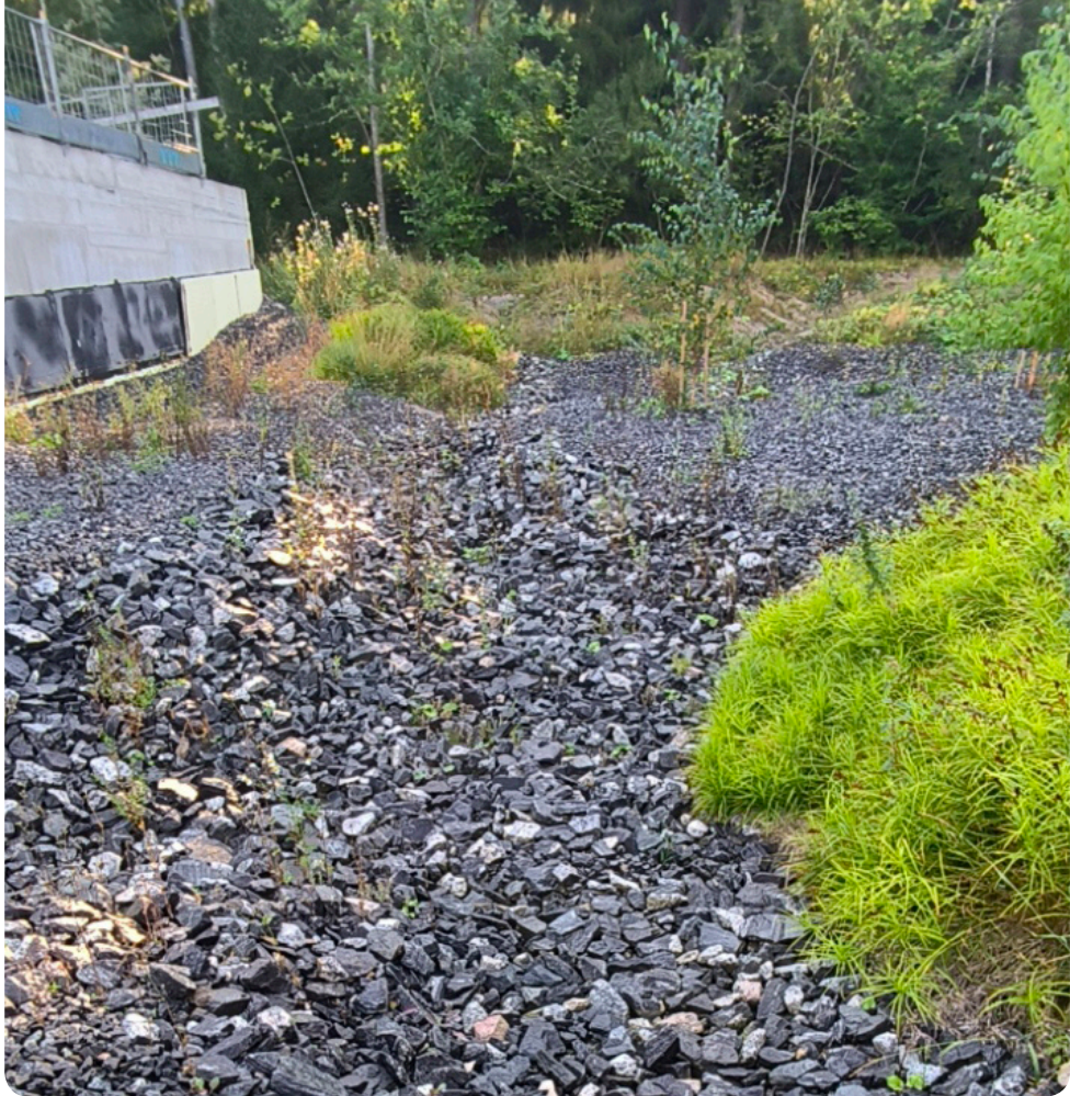
A soakaway consisting of stones of various sizes. Photo: Aleksi Reini
