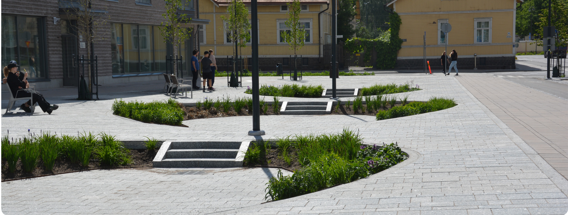
Depressions designed to collect floodwater have been created in the square in Kirstinpuisto, Turku. The area can be used for various recreational activities, such as skateboarding. Photo: Aino Saarinen
