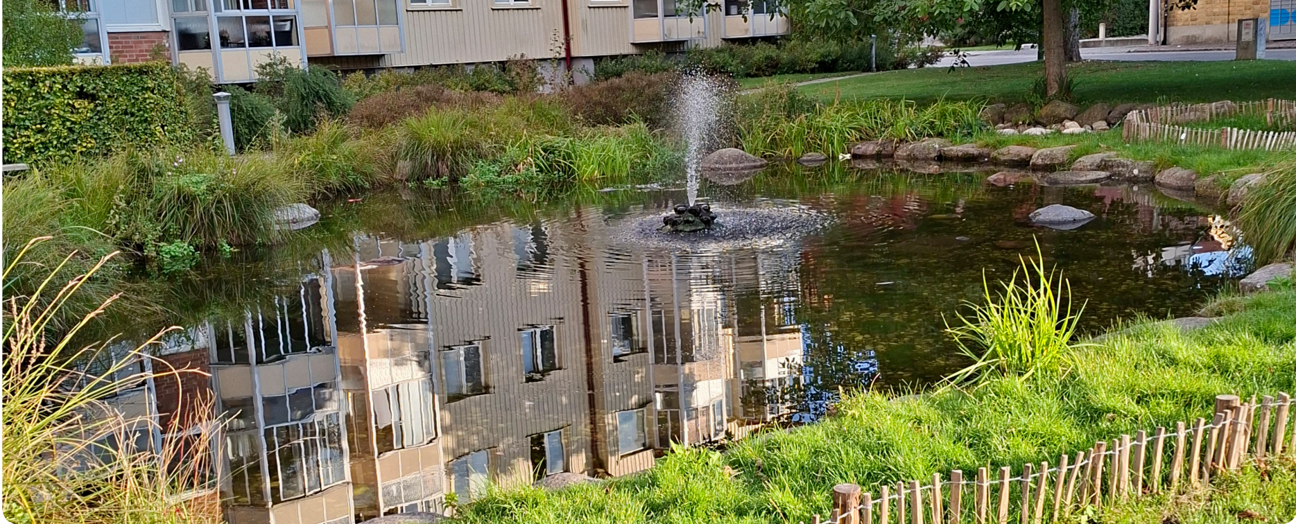
Nature-based stormwater management solutions have been successfully implemented in Augustenborg, Malmö, increasing the pleasantness of the neighbourhood and improving the area's image. Photo: Hilja Kurkinen
