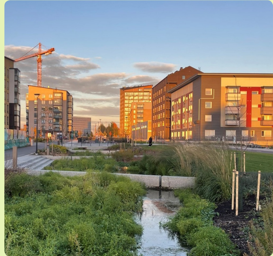
A stormwater swale in Kirstinpuisto, Turku, adds lush greenery to the urban landscape. Photo: Minna Kivimäki
