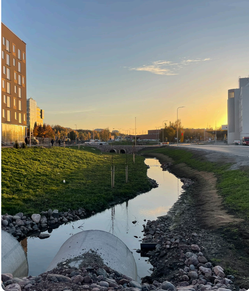
Two-stage channel at Saukonoja in Pukkila, Turku. Photo: Minna Kivimäki
