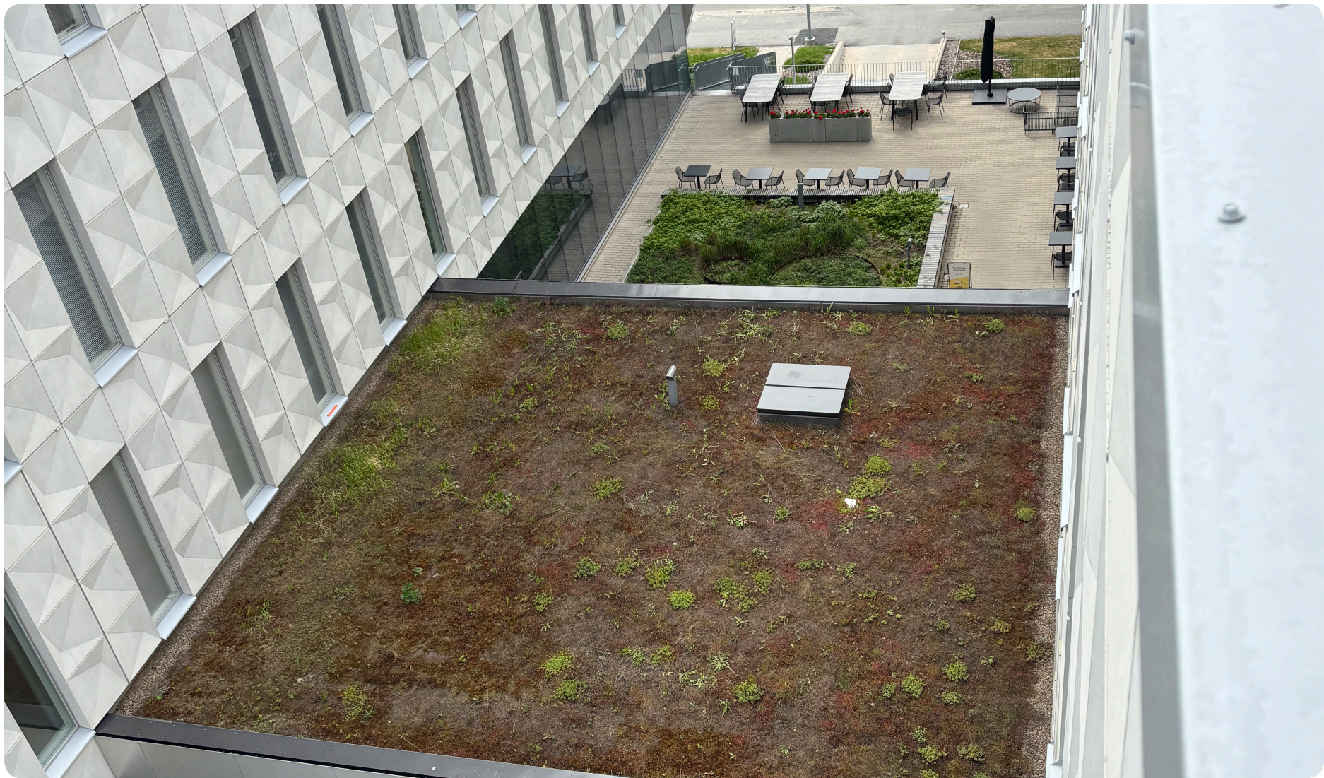
Turku Technology Properties has installed a small sedum roof at InfraCity. Photo: Turku Energia
