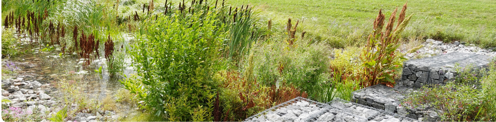
Filtration dam in a ditch. Photo: Minna Kivimäki
